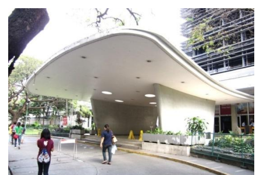
Building entrance canopy
