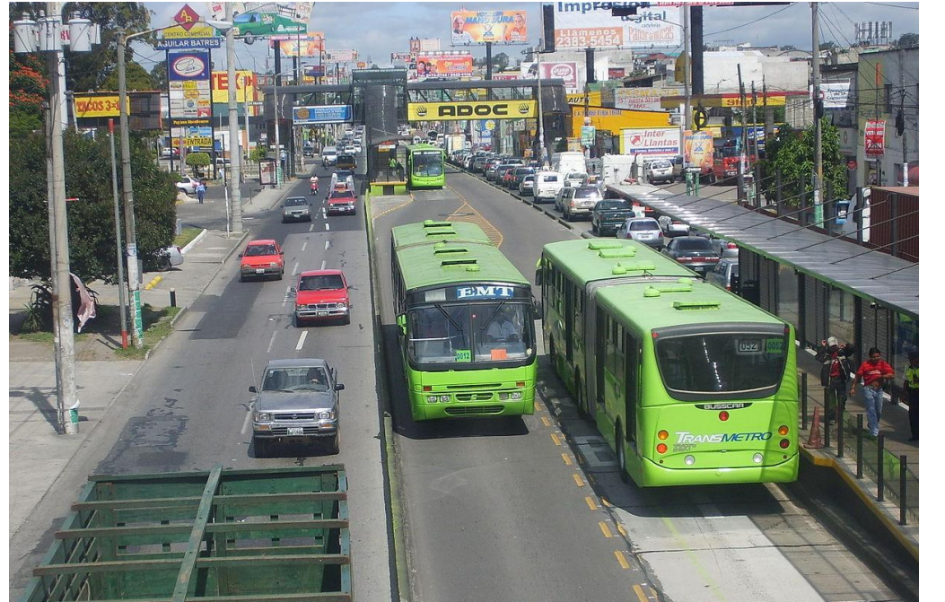
BRT corridor in intermediate phase
