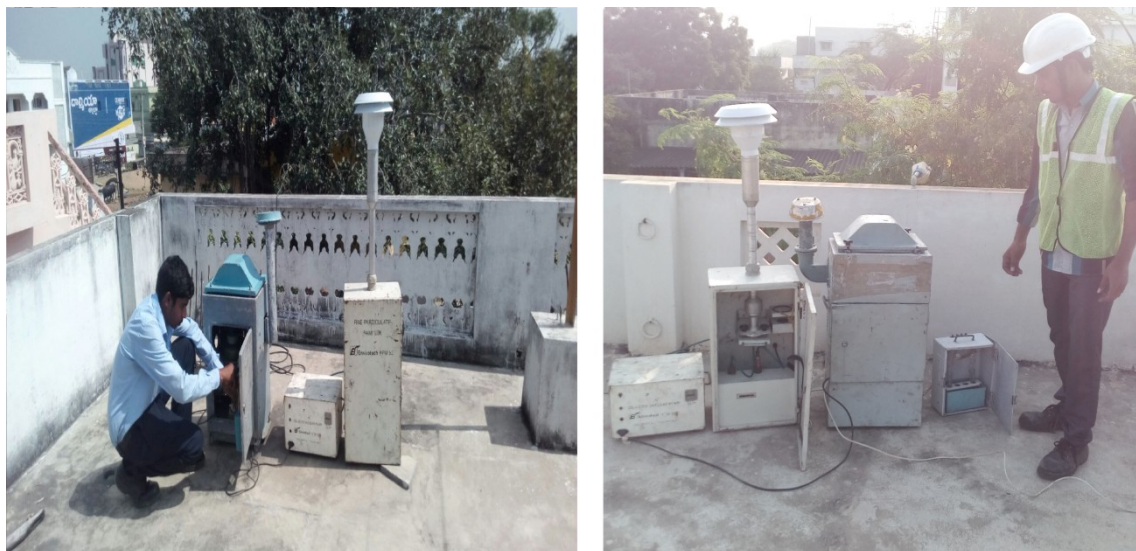
Figure 6-27 : AAQ Monitoring stations installed at Dondapadu and Navuluru
