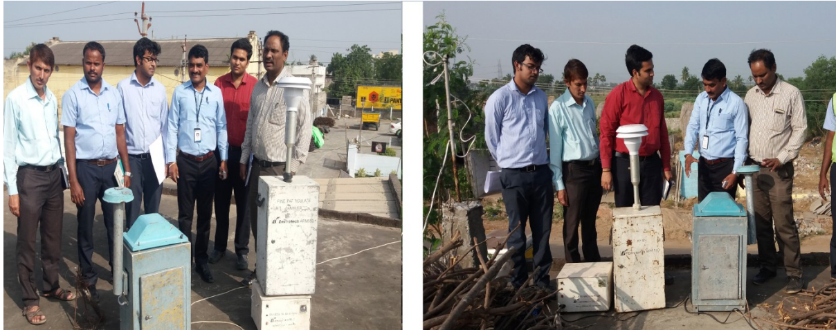
Figure 6-21 AAQ Monitoring stations installed at Malkapuram and Velgapudi
