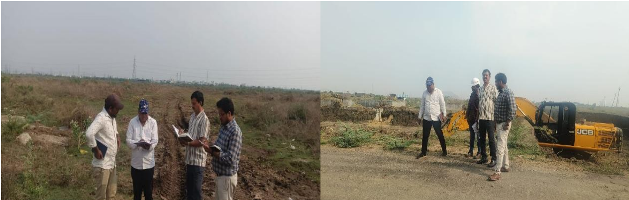
Zone – 3B & 5D Project sites are under cleaning & grubbing stage
