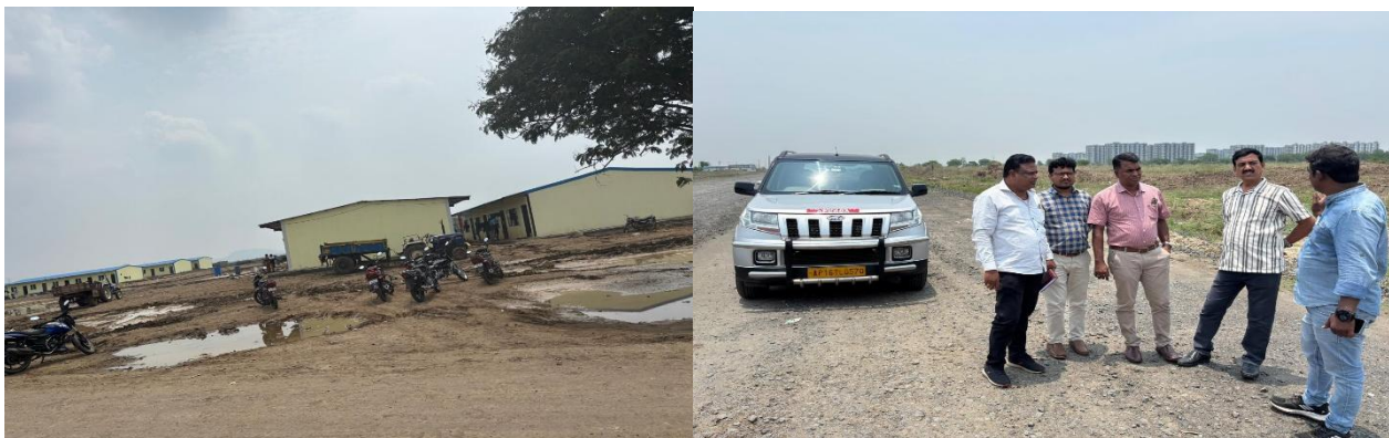
M/s RVR Labour Camp site at Thulluru Village
