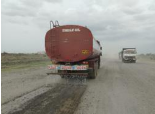
Figure 35: Dust control measures – Water sprinkling
