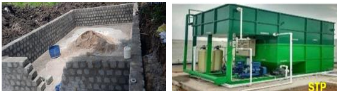
Figure 38: Sediment Tank and STP
