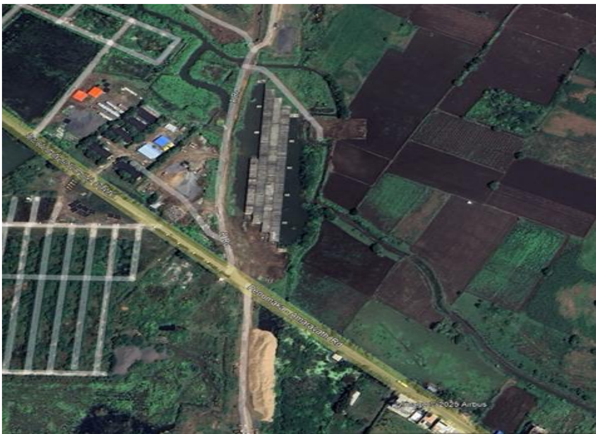
Figure 6-10: N4 Bridge Diversion Improvement for an Alternate route to Construction materials transportation
