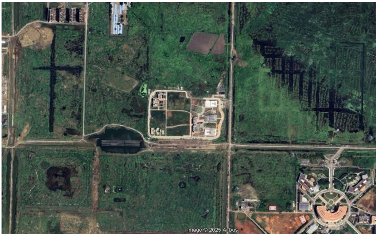
Figure 6-12: E8-N11 Bridge Diversion Improvement for an Alternate route to Construction materials transportation.
