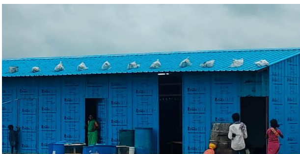
Figure 4-9: Placing sandbags on the roof of labour sheds
